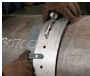
Adjusting for Guide Rail Overlap
