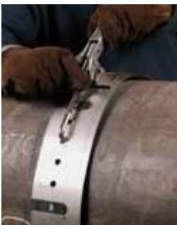
Clamping Guide Rail Overlap
